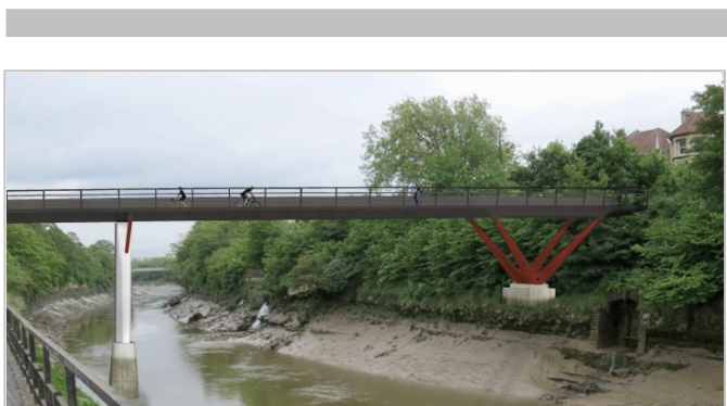
(a) Planning Application 14/04262/FB: New Camden Road Bridge (linking Coronation Road/Camden Road to Chocolate Path)
