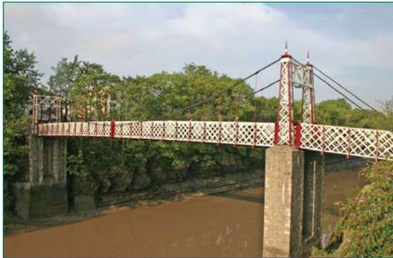
Gaol Ferry Footbridge
